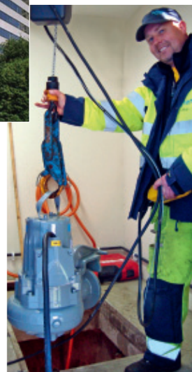
Right: Smart systems, like our new Flygt Expor pumping system and SmartRun control system, are the wave of the future for wastewater facilities.
