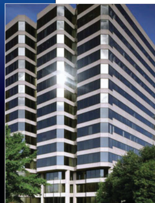
"Green" buildings, like the Monarch Plaza in Atlanta, Georgia, use our energy- and water-saving products to meet international efficiency standards.
